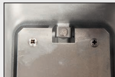
Internal earth screw in body
